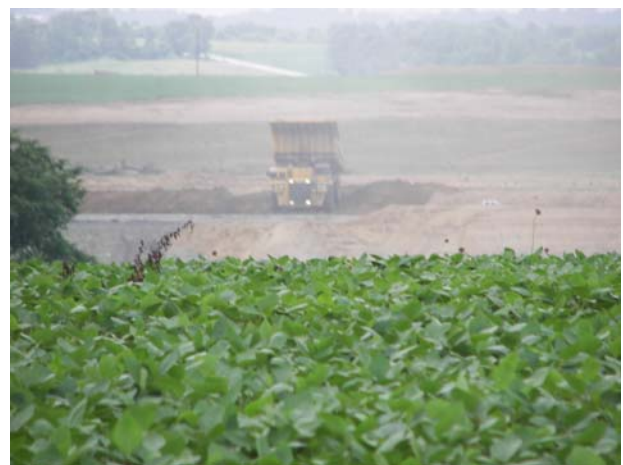
Soil being replaced as part of the reclamation process. Photo courtesy of Peabody Coal
