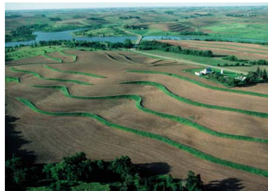
Terraces installed in a crop field to slow runoff and reduce erosion.
