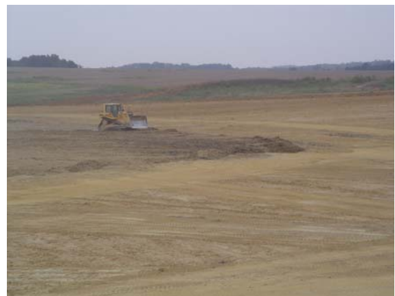
Topsoil being replaced on subsoil material. Photo courtesy of Peabody Coal
