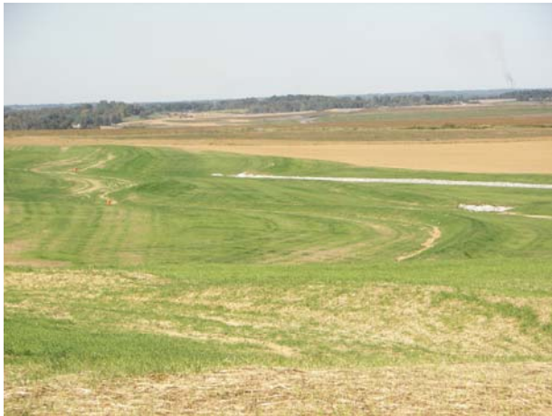
Contours used to control water on reclaimed land. Photo courtesy of Peabody Coal
