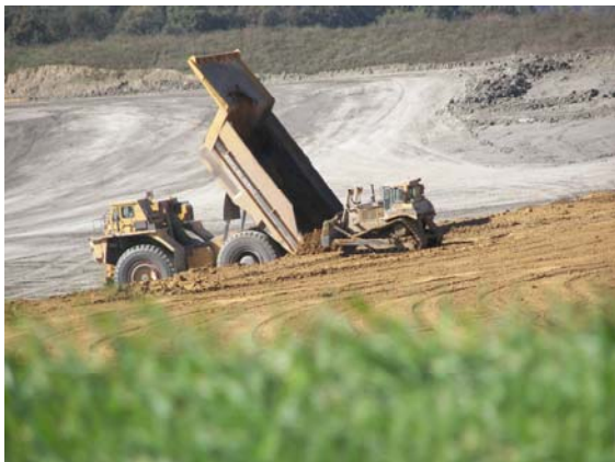
Soil material being replaced over graded spoil as part of the land reclamation process. Photo courtesy of Peabody Coal
