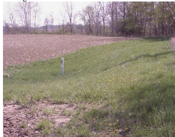
WASCOB embankment (right) and riser for drainage
