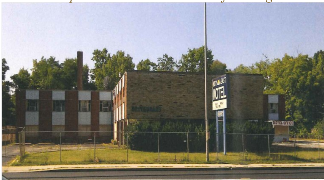
Before: Former Indy East Motel, 5585 East Washington Street
