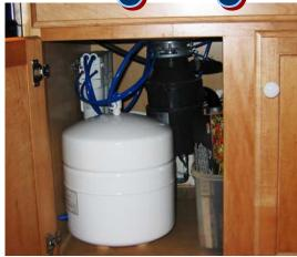
At the Glenn Hills Non Profit Water Corporation, each residential point-of-use system is comprised of a recharge tank and filtration unit (situated behind the recharge tank), which easily fits under the kitchen sink.
