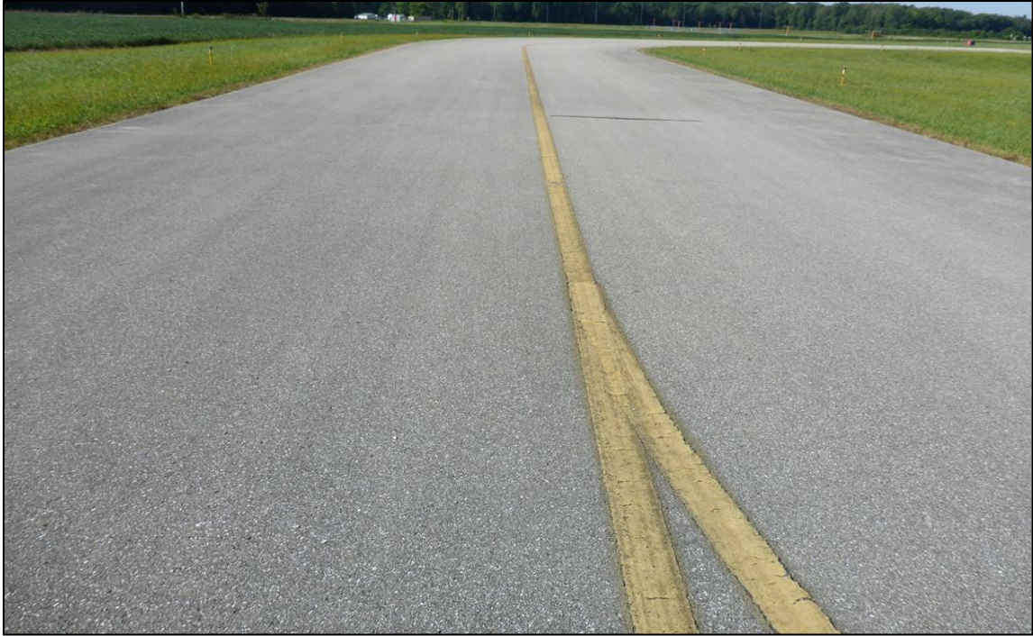
Figure 2-4. Typical AC Pavement in Good Condition (Feature 120)
