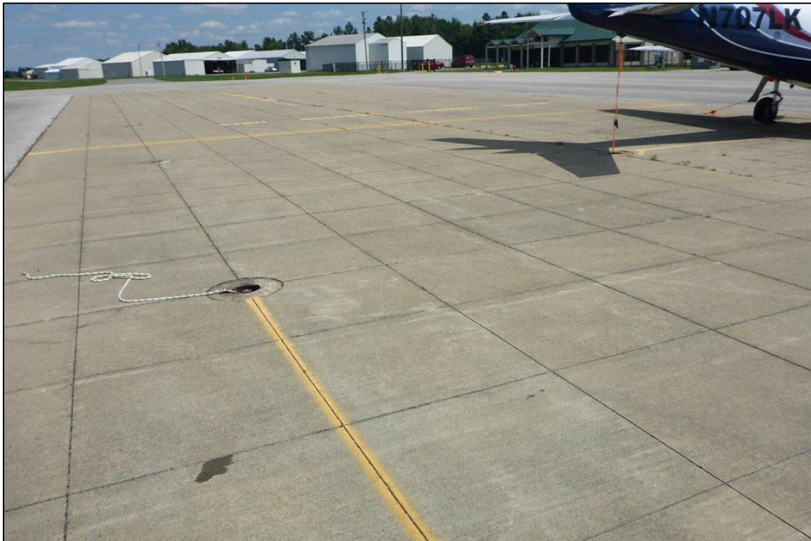
Figure 2-3. Typical PCC Pavement in Good Condition (Feature 3020)
