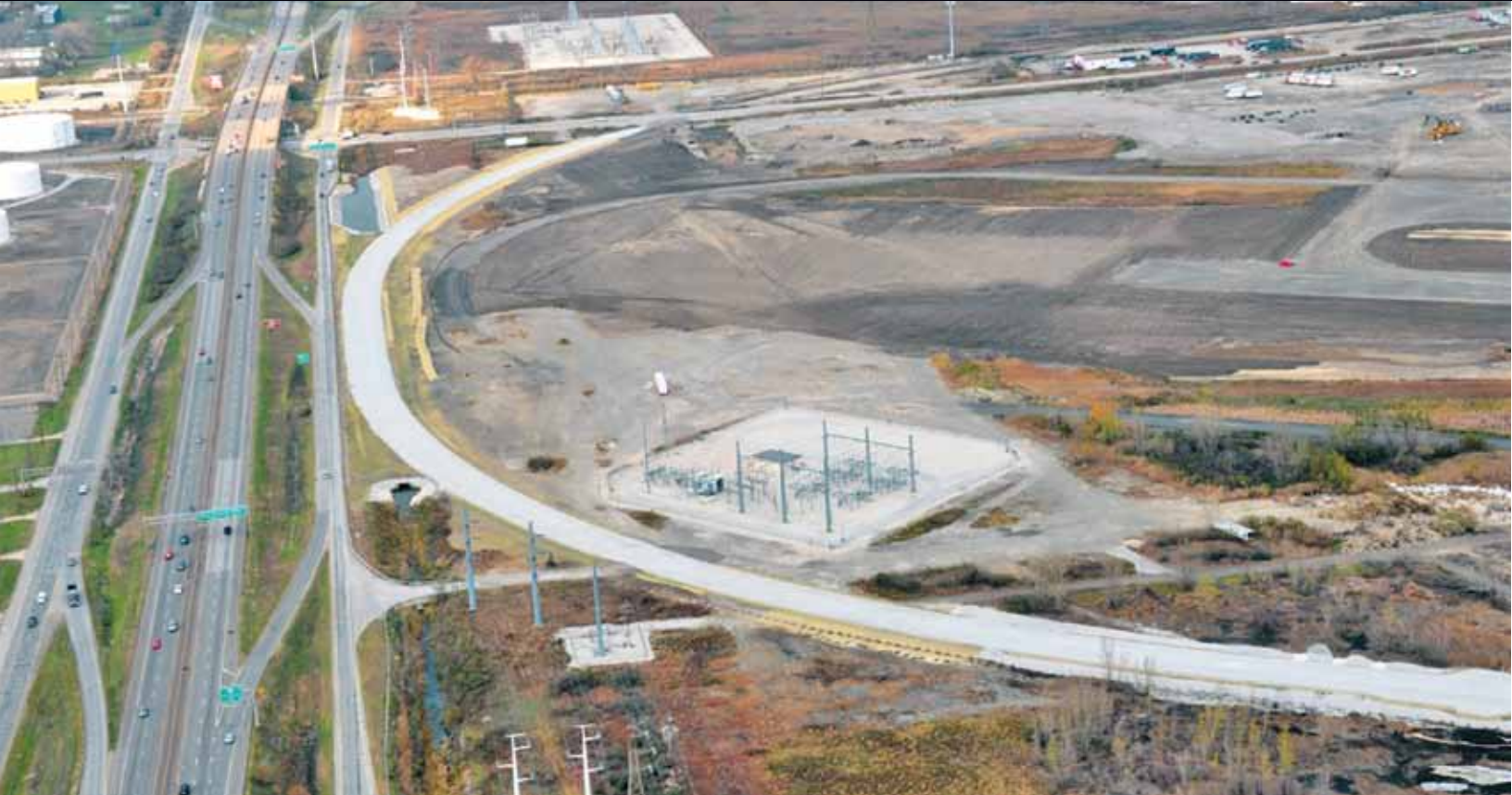
The finished culvert, topped by the new rail bed, in November 2012.
