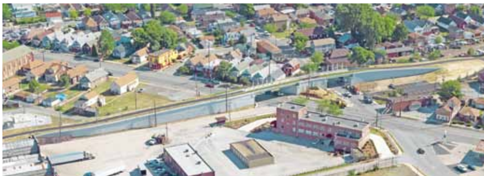
Passing over busy Indianapolis Boulevard, the new $4 million George Lake Pedestrian Bridge opened in May 2012. It is a critical link in the Marquette Plan's vision for a trail system running the length of the Lake Michigan shoreline in Northwest Indiana, and connecting to the waterfront trails in Chicago. In October, the Indiana Metropolitan Planning Organization Council honored the bridge with a 2012 Outstanding Transportation Project award in the category of Special Design or Construction.
