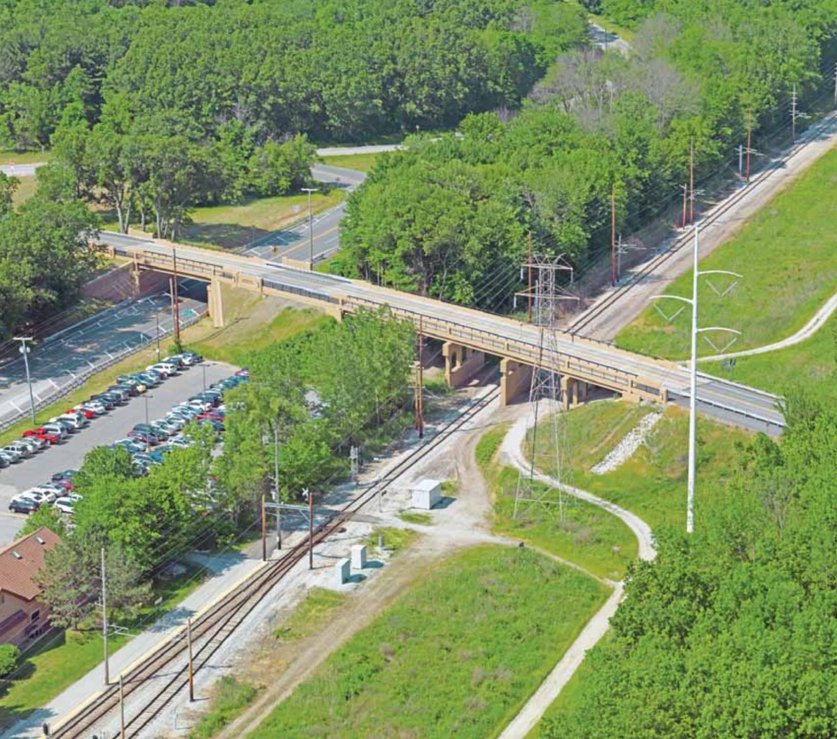
The new U.S. 12 bridge at the South Shore's Dune Park station in Chesterton.
